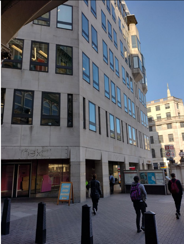
Charing Cross station forecourt frontage
